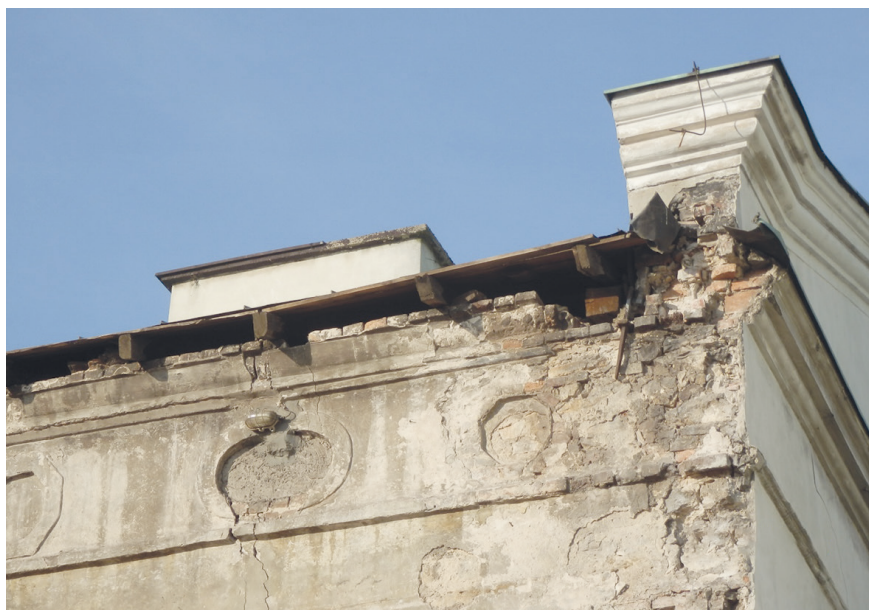
Fig. 10. Exposed drawing of the cornice together with the architectural detail of the historic monastery building. Photo by M. Błażewicz
