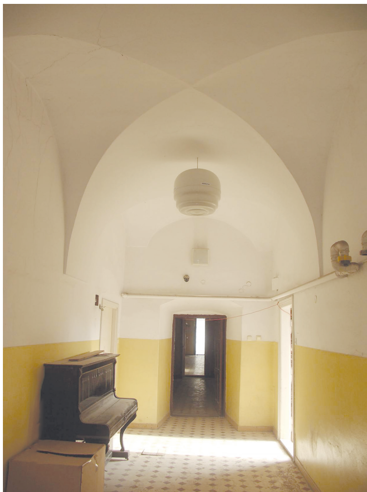
Fig. 23. Suspended from the vault, the device uses the gravitational field and the earth's magnetic field to stop capillary rise of water from the ground. Photo by M. Błażewicz
