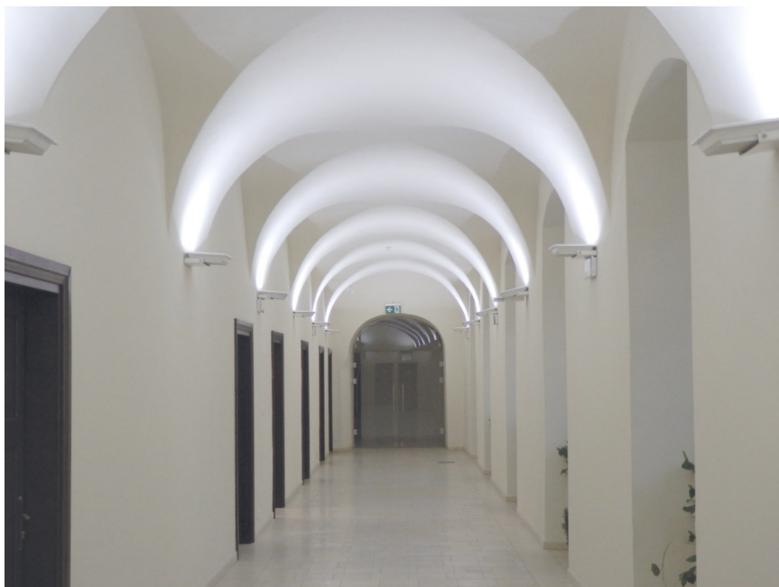
Fig. 15. The south wing of the monastery was added in 1729; the corridor is covered with barrel vaults with lunettes. Photo by M. Błażewicz
