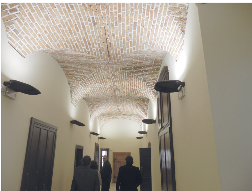
Fig. 14. The corridor tract on the east side was added in the 17 th century. Wooden ceilings were replaced with brick cross vaults. In the realisation, the vault contrasts clearly with the walls to emphasise the difference in the time of their creation. Photo by M. Błażewicz
