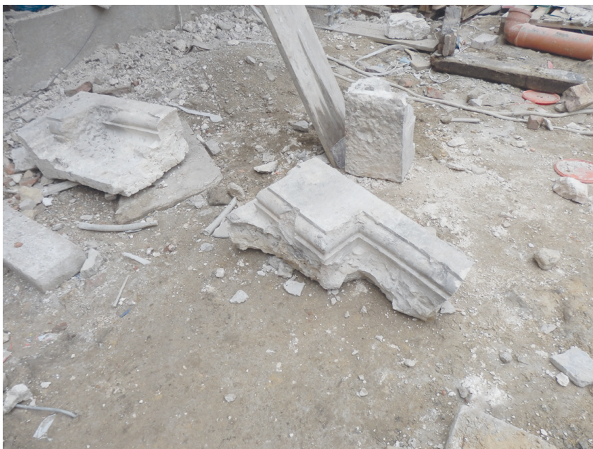
Fig. 13. Fragments of a stone window band. These elements were found in the stone wall structure of the building. They served as building material in the next phase of construction. Photo by M. Błażewicz
