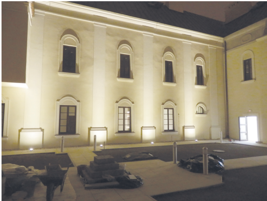
Fig. 18. The southern wing of the monastery, the reconstruction of the 18 th century remnants of pilasters and the introduction of simple window frames. Photo by M. Błażewicz
