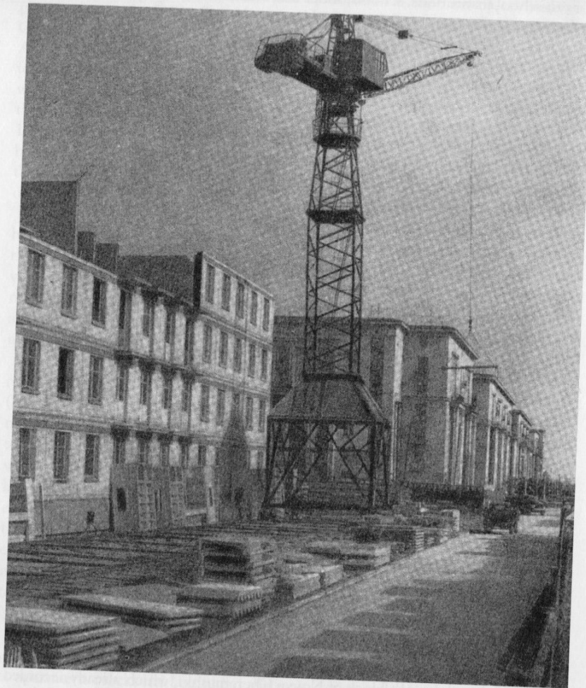
Figure 10.1 Assembly of a large-panel apartment house on Block 123 of Ivanovskaya Ulitsa in the Neva District of St Petersburg. Photograph from the magazine Arkhitektura SSSR , 1958, No. 1, p. 30.
