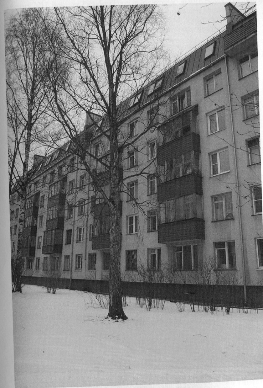
Figure 10.4 Apartment house of the 1-LG-507 series. 16, Torzhkovskaya ulitsa, Saint Petersburg. Reconstructed in 1999–2001. Photograph by D. Liubimova, 2017.
